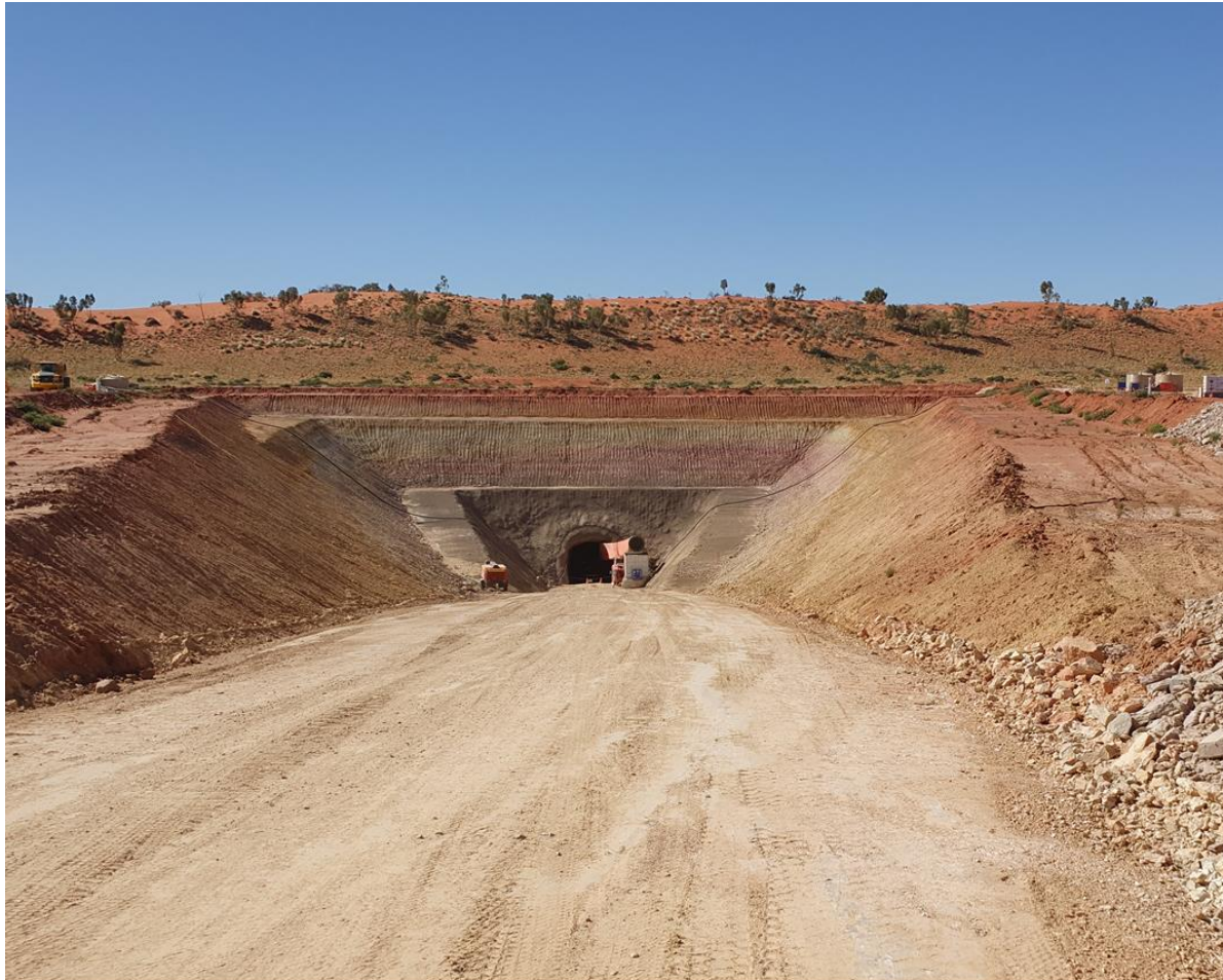
Havieron Exploration decline has advanced 189 metres as at 29 September 2021
