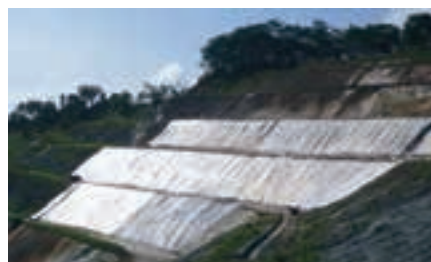
FIGURE 7: GOSOWONG PIT REHABILITATION AND DRAINAGE MANAGEMENT
